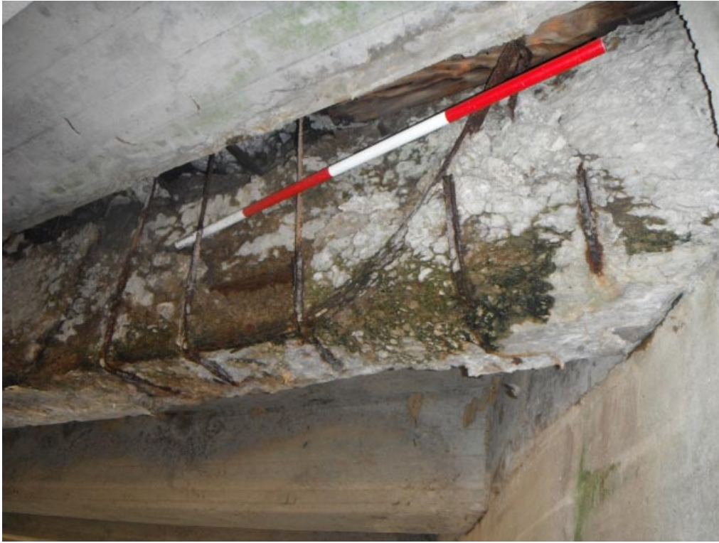
Beam 3 at the south end near the south abutment (A1) has severe deterioration and resteel with 100% section loss.
