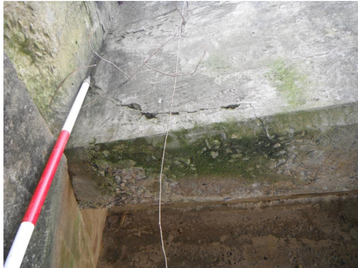
Beam 7 east face near the south abutment (A1) has cracking and deterioration.
