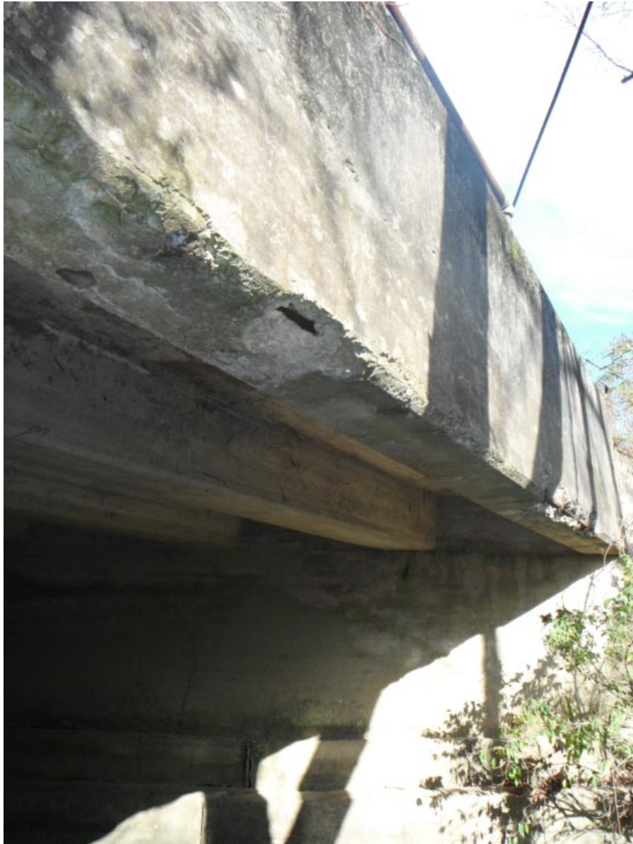
East side looking north at spalling on bottom of beam 7.
