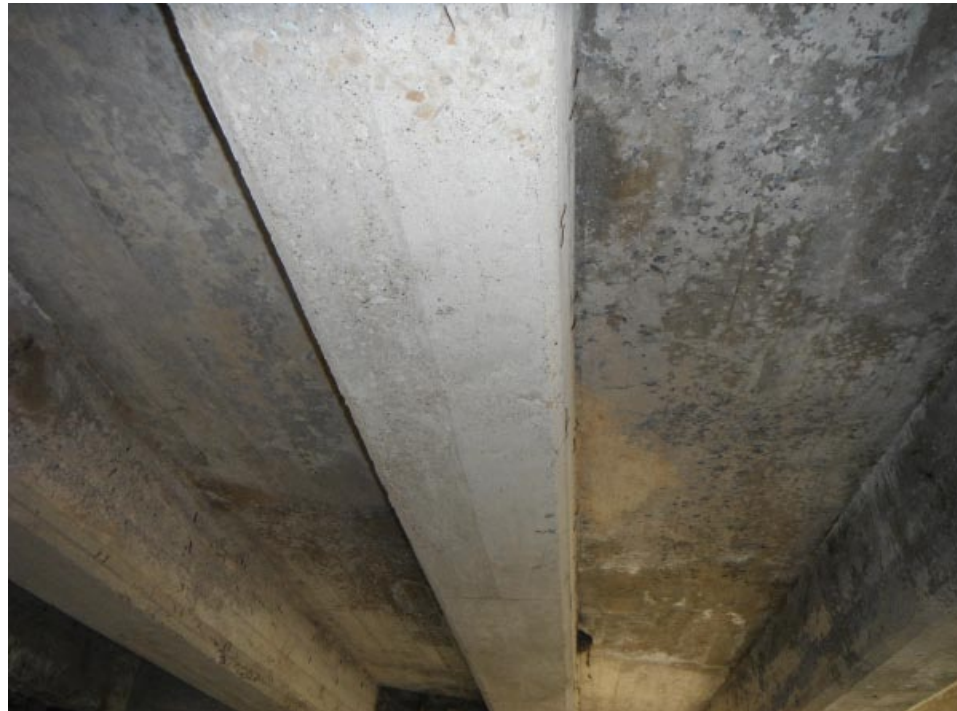
Soffit of bays 4 and 5 looking north.
